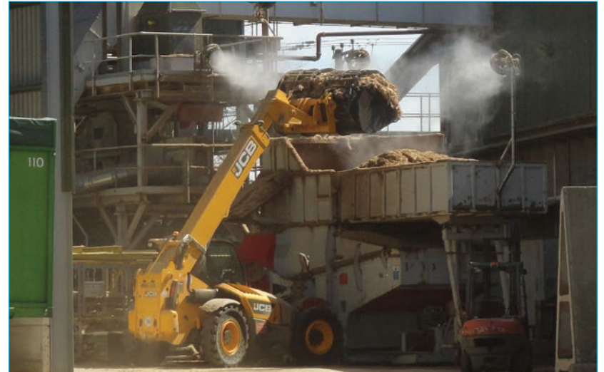
Biomass Woodchip Storage
