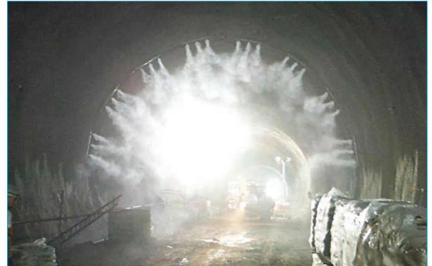
Tunnelling for the new tube lines under London & Edinburgh
